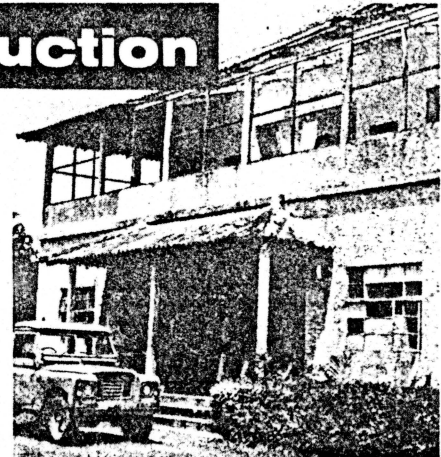
ADMINISTRATION headquarters in Lunbo district, Zambezia province, destroyed by bandits.
