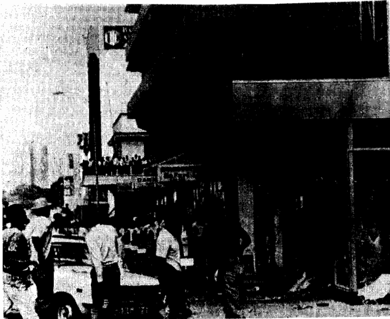
SMOKE pours out of the SAA offices in Union Avenue yesterday.
