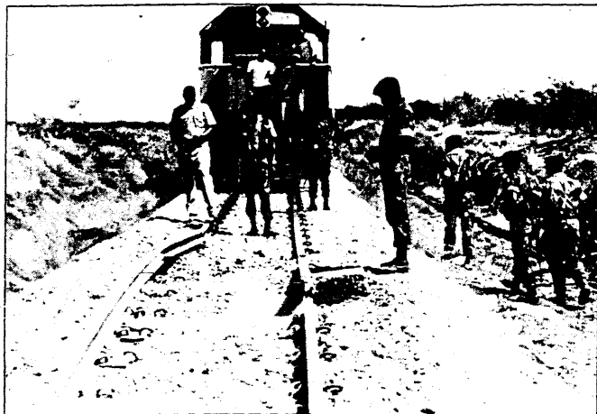
The destruction of physical infrastructure has made it difficult to move supplies to inland centres
